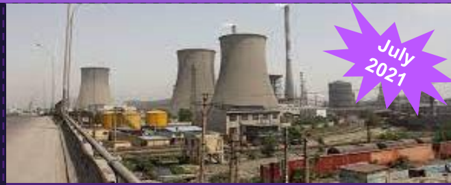
525 MW IPP – East India
